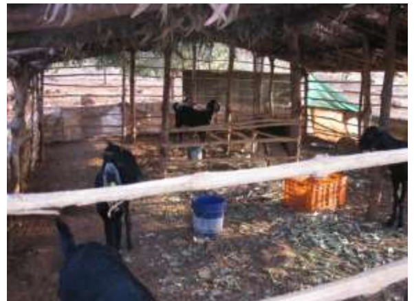
Newly built goat shed by a beneficiary tribal farmer ( Gawandh village)
