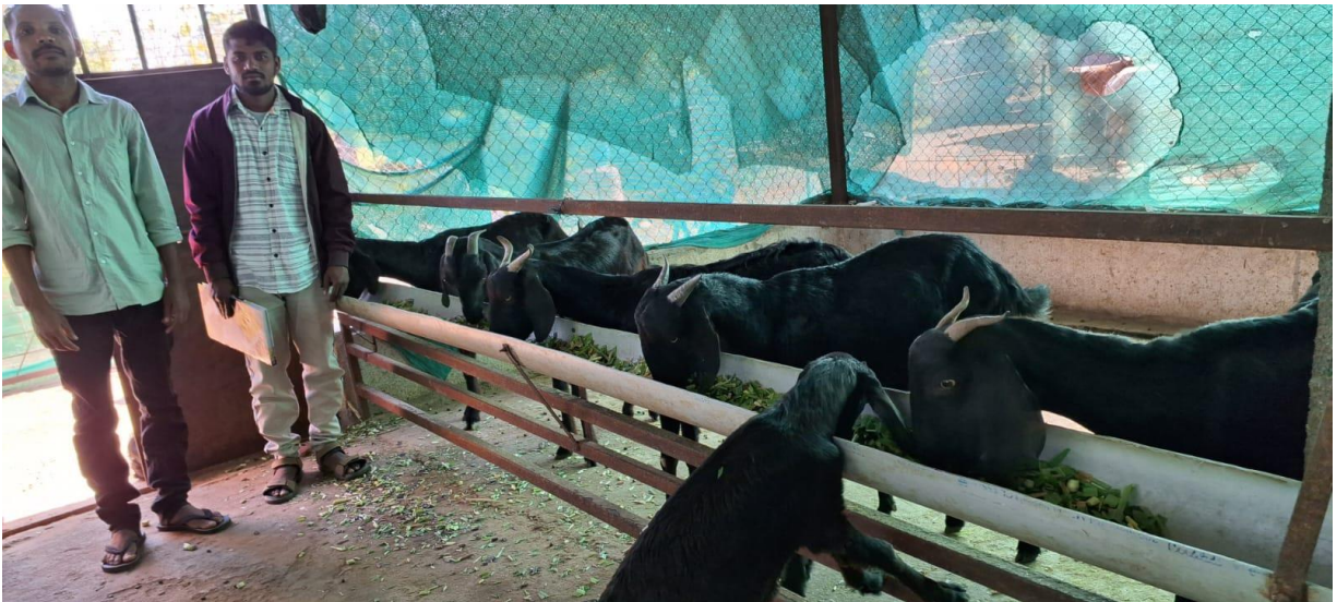
A farmer constructed new goat shed with concrete, wire mesh, shed net wall & GI sheet roof along with metallic feeder
