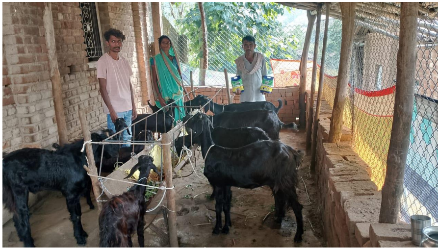
A low-cost shed made by GI wire mesh, brick with earthen floor and metallic feeder
