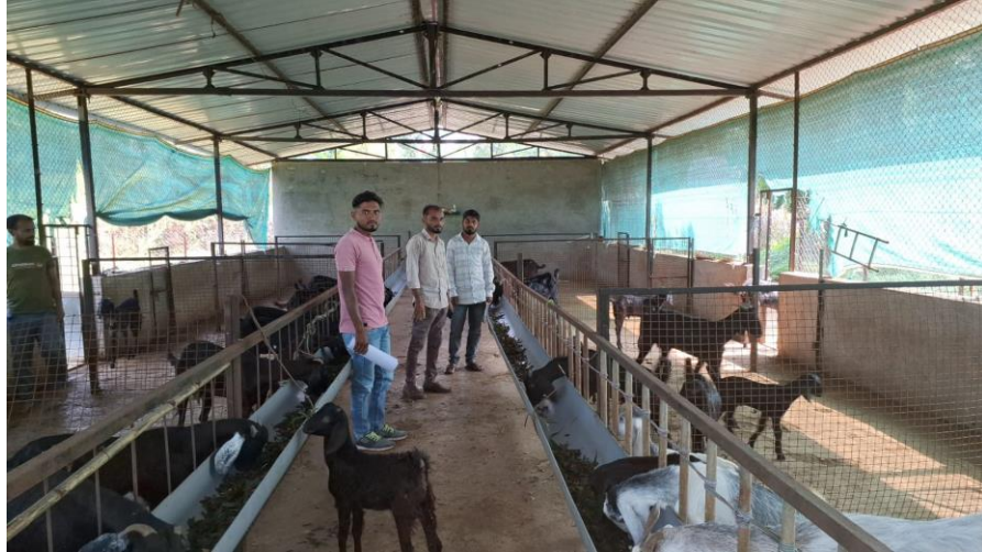
RCC shed having GI sheet roof, concrete floor and wall with metallic feeder
