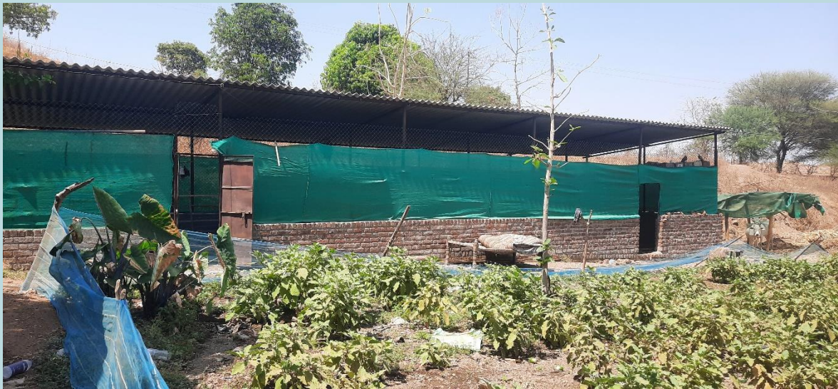
A newly constructed goat shed by one of the beneficiary farmers
